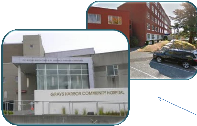
Grays Harbor Community Hospital
